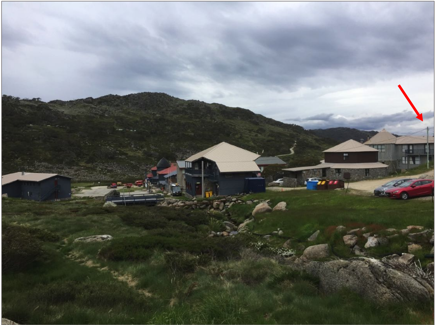
Figure 4. The subject utility pole (as indicated by red arrow) proposed to host telecommunications equipment in context to the surrounding terrain and buildings (view North).
