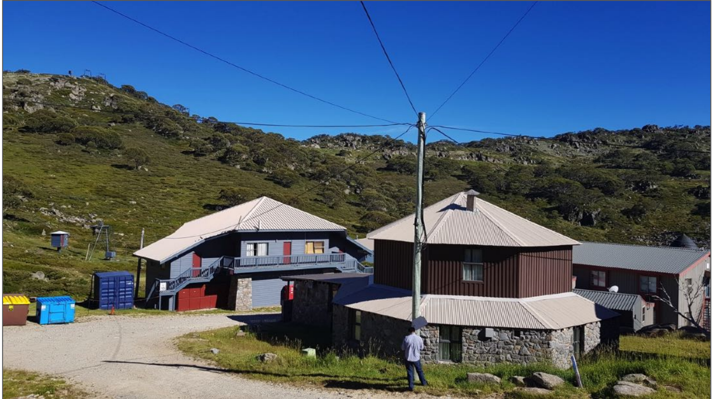
Figure 10. The existing timber pole and surrounds
